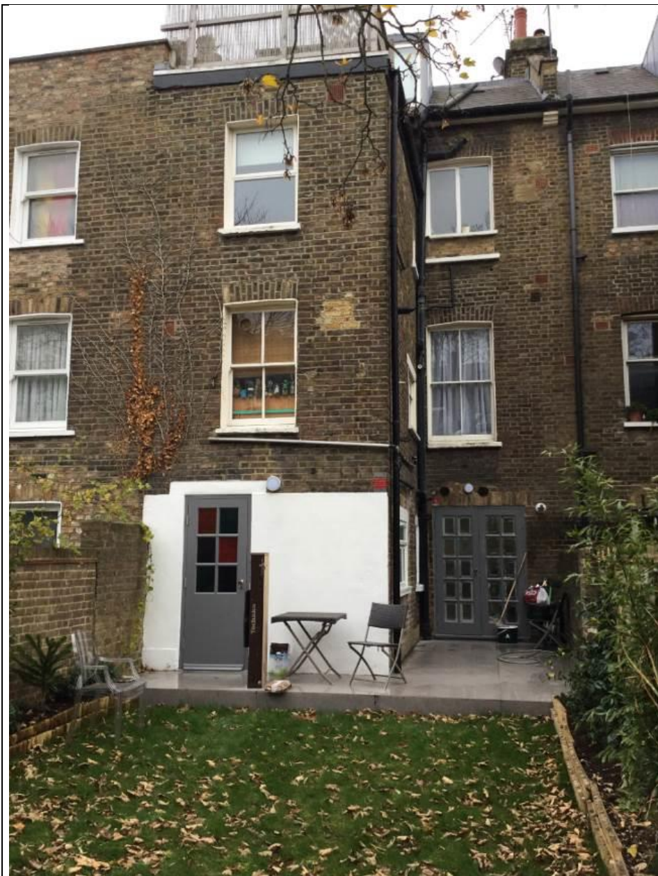
Rear Elevation of 245 Shirland Road
